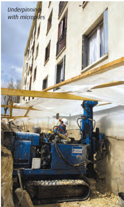
Underpinning with Fondapieu
