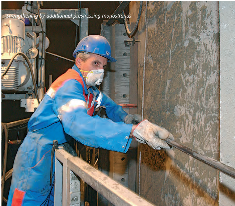
Columns repair by shotcreting
