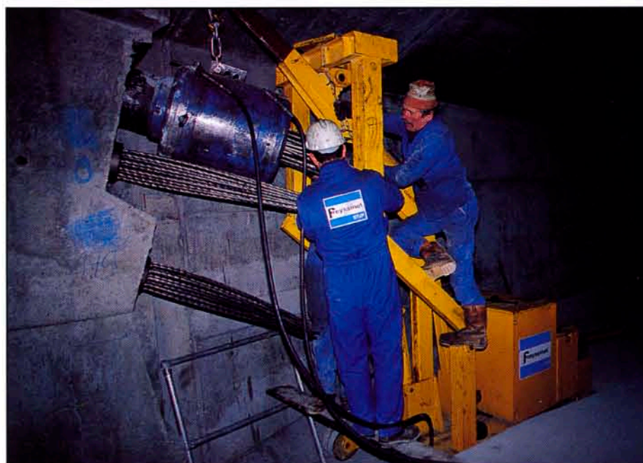
Meys siez TGV Viaduct: tensioning operations
