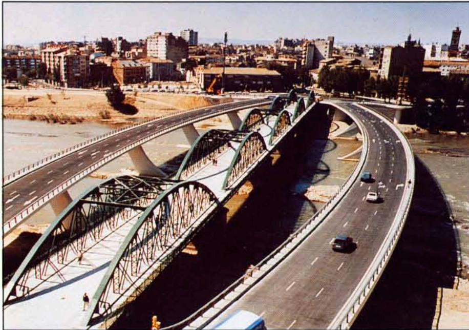
Pilar Bridge: general view
