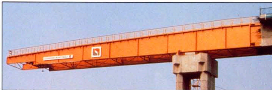
Jules Verne Viaduct - Amiens: launching nose
