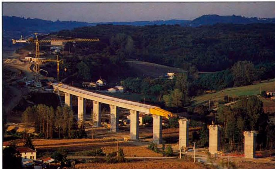
Meys siez TGV Viaduct: general view
