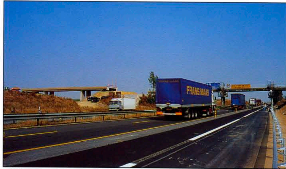
A1 Motorway: overpass 135
