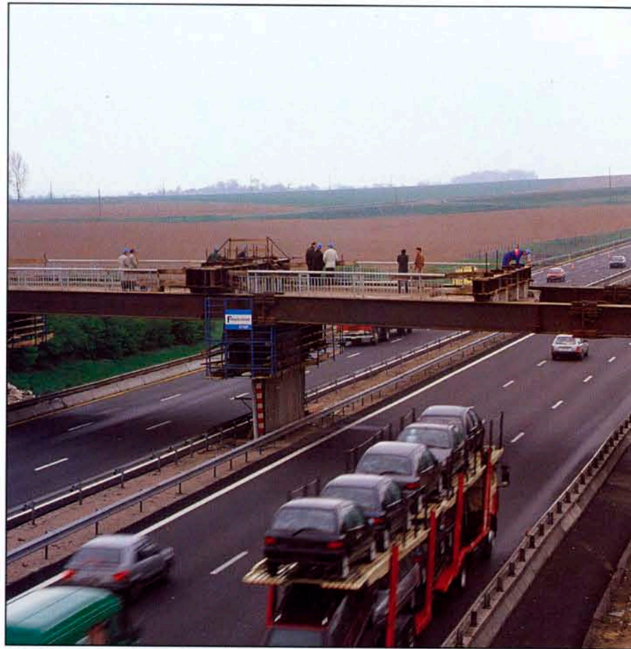
A1 Motorway: demolition of overpass 106
