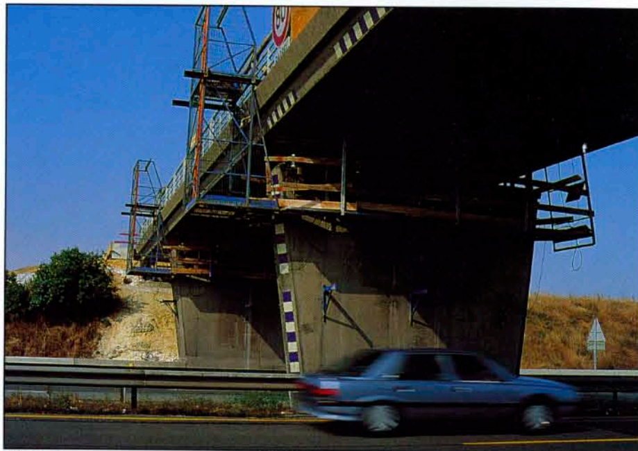
A1 Motorway: overpass 135 scaffolding
