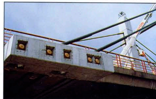
Overpass 73 stay cable deck anchorage...
