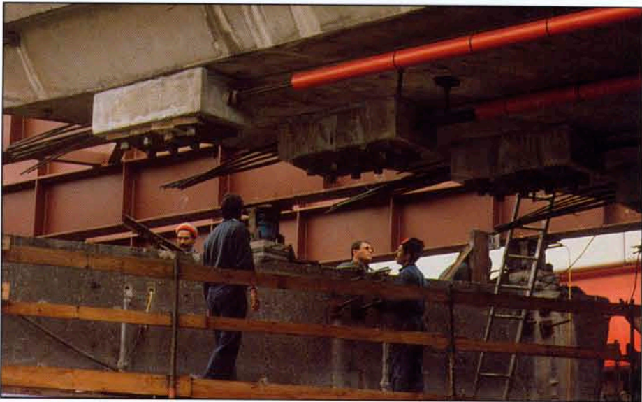
A7 Motorway: Reventin-Vaugris overpass demolition
