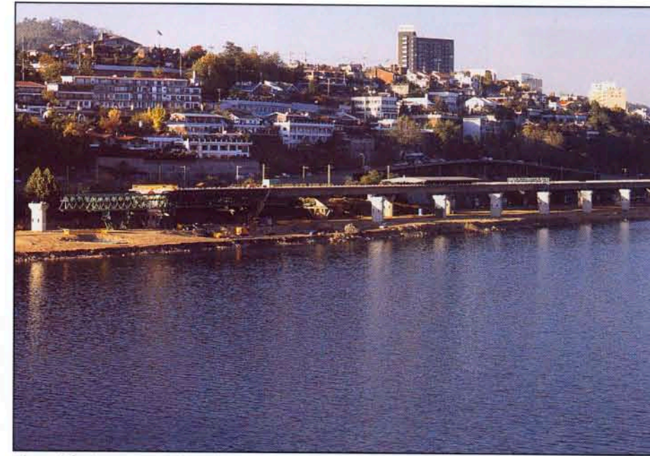
Riverside I: construction site
