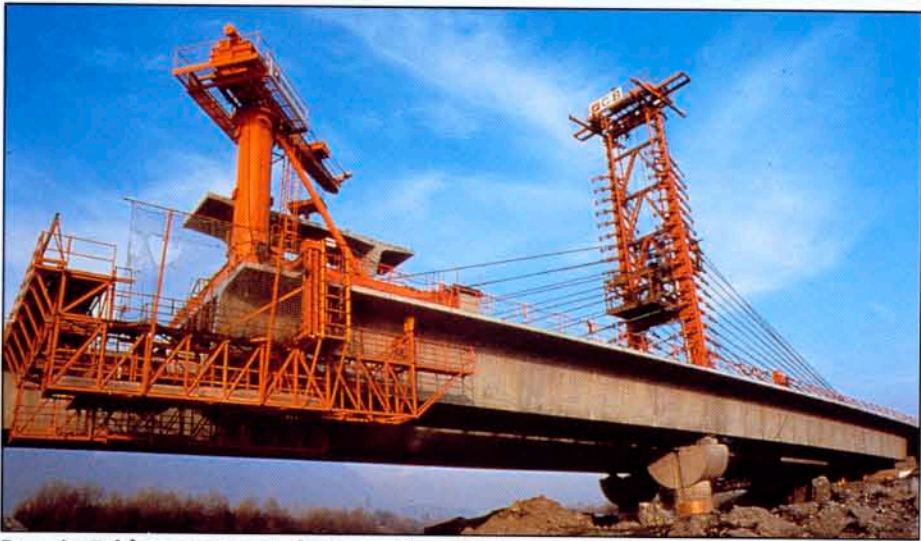
Francin Bridge: segment placing with swivel crane
