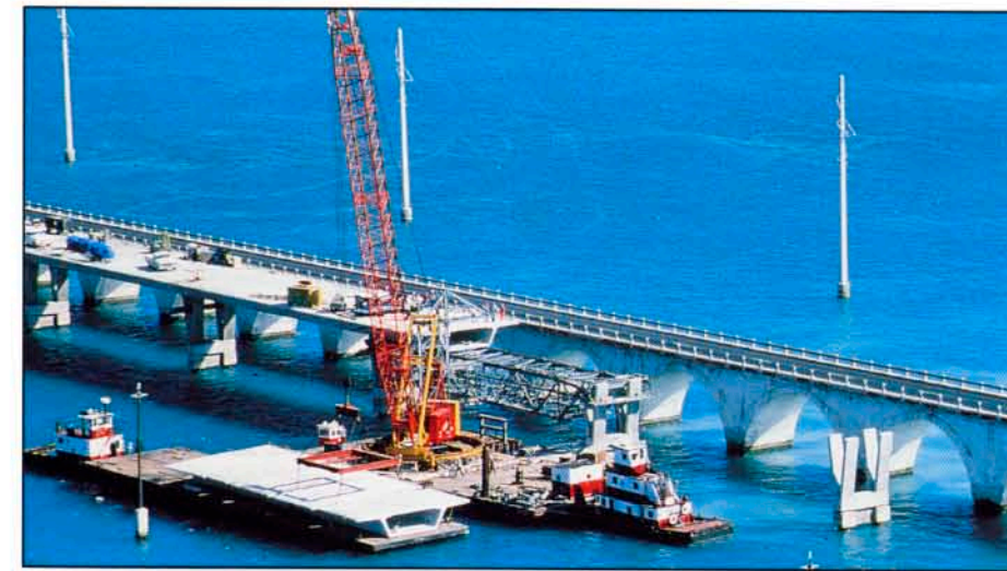
Long Key Bridge: construction site
