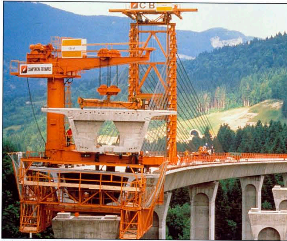
Frebuge Bridge: staying mast and swivel crane
