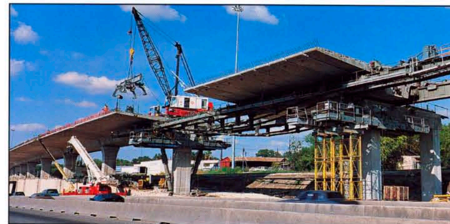
San Antonio Viaduct assembly truss
