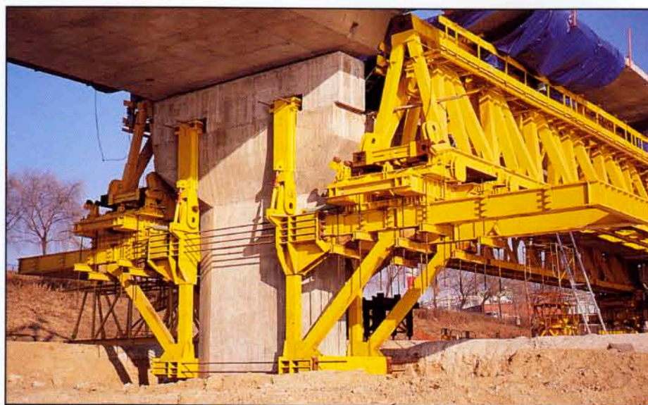
Riverside IV: assembly truss and pier segment
