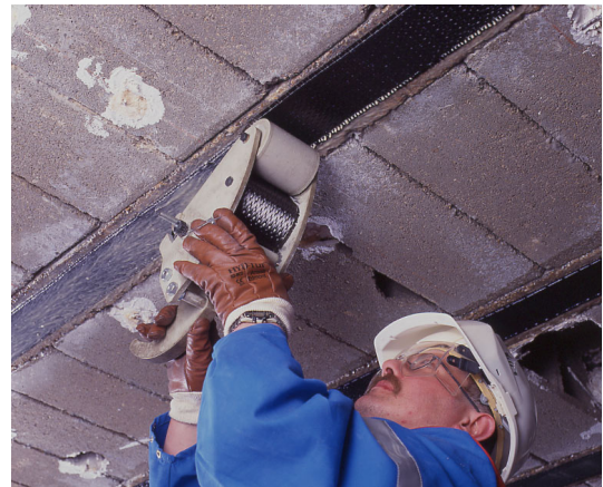
Application of the carbon fabric
